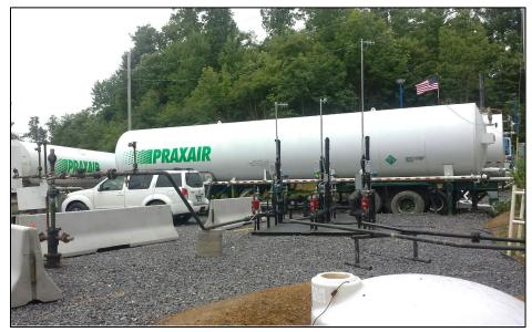
Figure 3.5: Injection operations at the DD-7 well pad. Background: CO<sub>2</sub> storage tanks. Middleground: Injection skid. Foreground (Left): DD-7 wellhead. Foreground (Right): Pipeline to DD-7A and DD-8.
