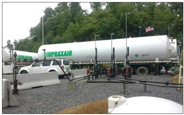
Figure 2.12: Injection operations at the DD-7 well pad. Background: CO<sub>2</sub> storage tanks. Middleground: Injection skid. Foreground (Left): DD-7 wellhead. Foreground (Right): Pipeline to DD-7A and DD-8.
